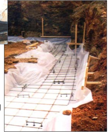
Plastic wrapped beneath footing
